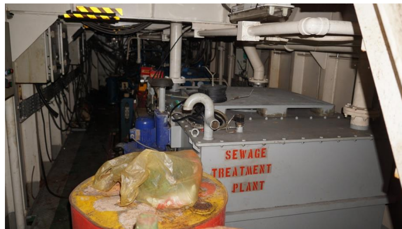
Sewage Treatment Plant
